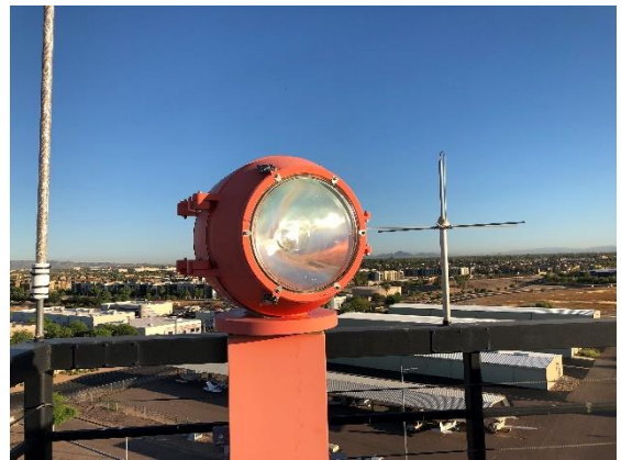
Figure 3: Beacon Light at top of ATCT
